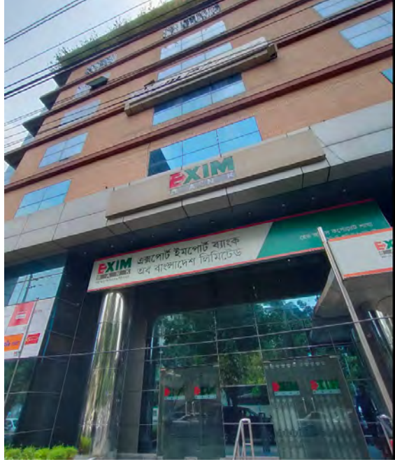
Figure 3.1:Bank Head Office
