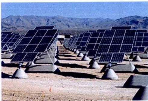
1.1.4 Figure: Tilted axis sun tracker
