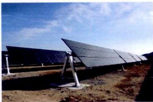
1.1.3 Figure: Horizontal axis sun tracker
