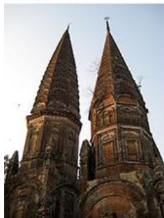
SONARONG TEMPLE, BRICK & STUCCO MASONRY
