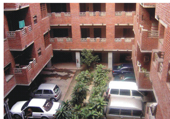
Figures 2 & 3: Recent courtyard type buildings
