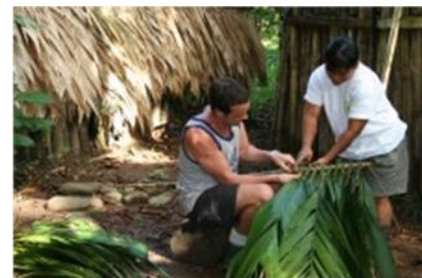
Fig: Local techniques of making roof with palm leaves
