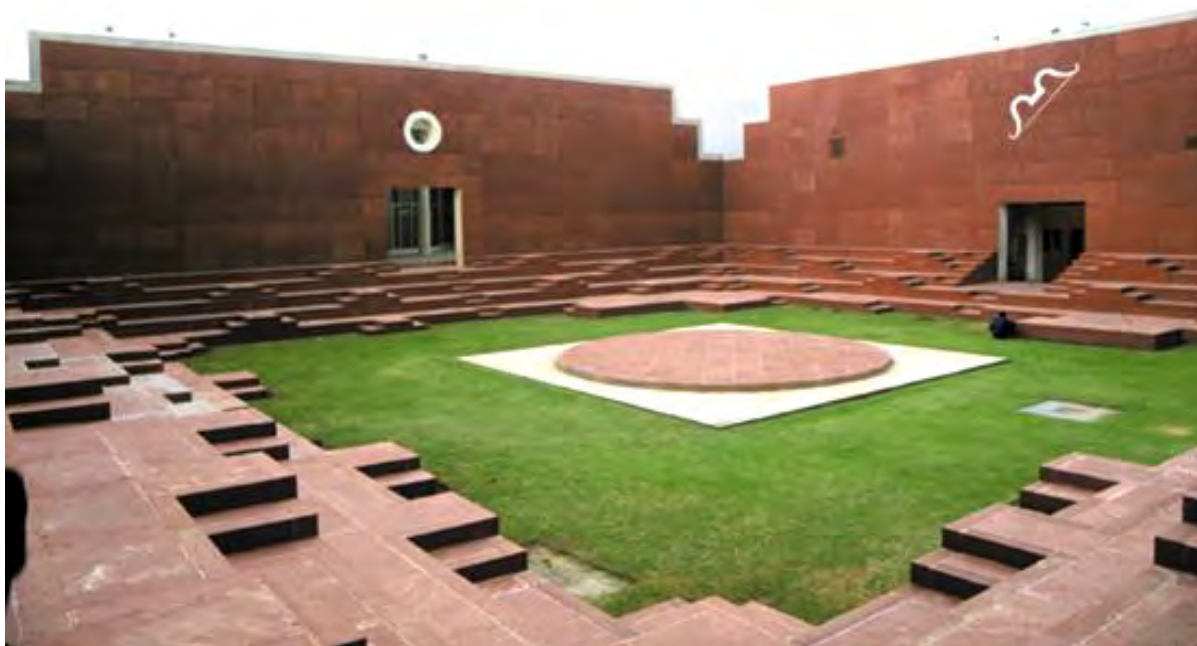
Fig-18 Central courtyard of Jawahar Kala Kendra
