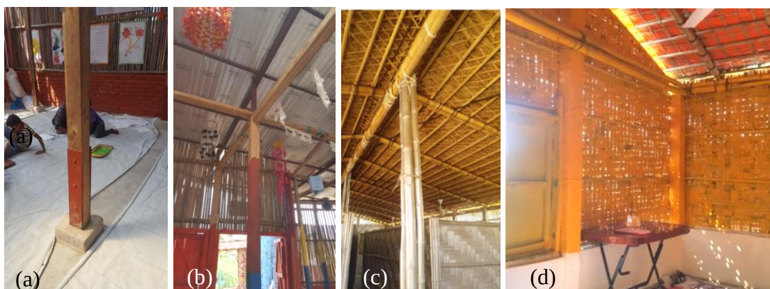
Figure 21: Images of structural material. Image (a), (b) shows wooden column-beam, (c) shows bamboo column beam, (d) shows precast column and bamboo beam. Source: Field survey by Author, 2020
