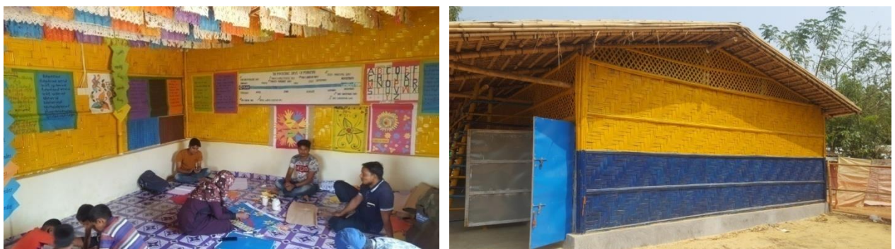
Figure 19: Images of wall material. Image (a) shows the wall made of brick and bamboo, Image (b) shows the wall made completely with bamboo. Source: Field survey by Author, 2020
