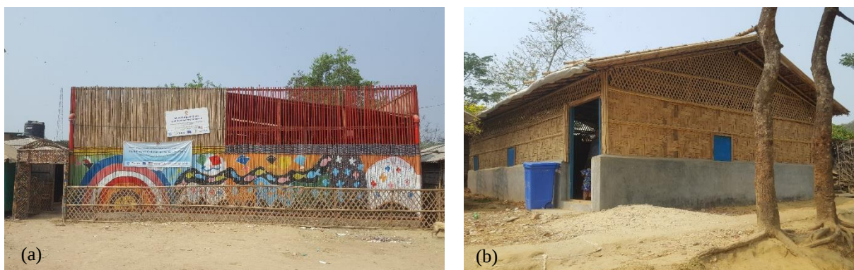
Figure 26: CFS designed by different agencies. (a) Image of a CFS designed by an expert team, (b) Image of a CFS designed by an agency following a layout by funding agencies.
