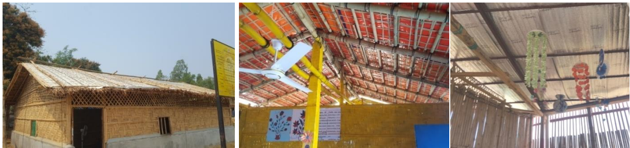
Figure 20: Images of roof material. Image (a) and (b) shows thatch roof with tarpaulin on both, image (c) shows roof of CI sheet with metal purlin and thermal insulator. Source: Field survey by Author, 2020
