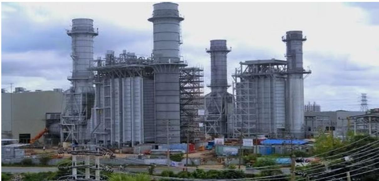
Fig. 4.7 450 MW CCPP (North) Plant
