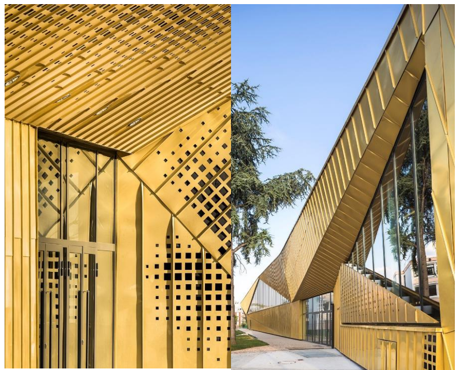
Figure 27: Façade details of the complex
