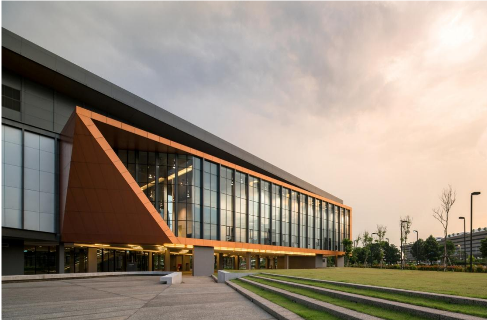
Fig.4.2.2: CAT Telecom Headquarter
