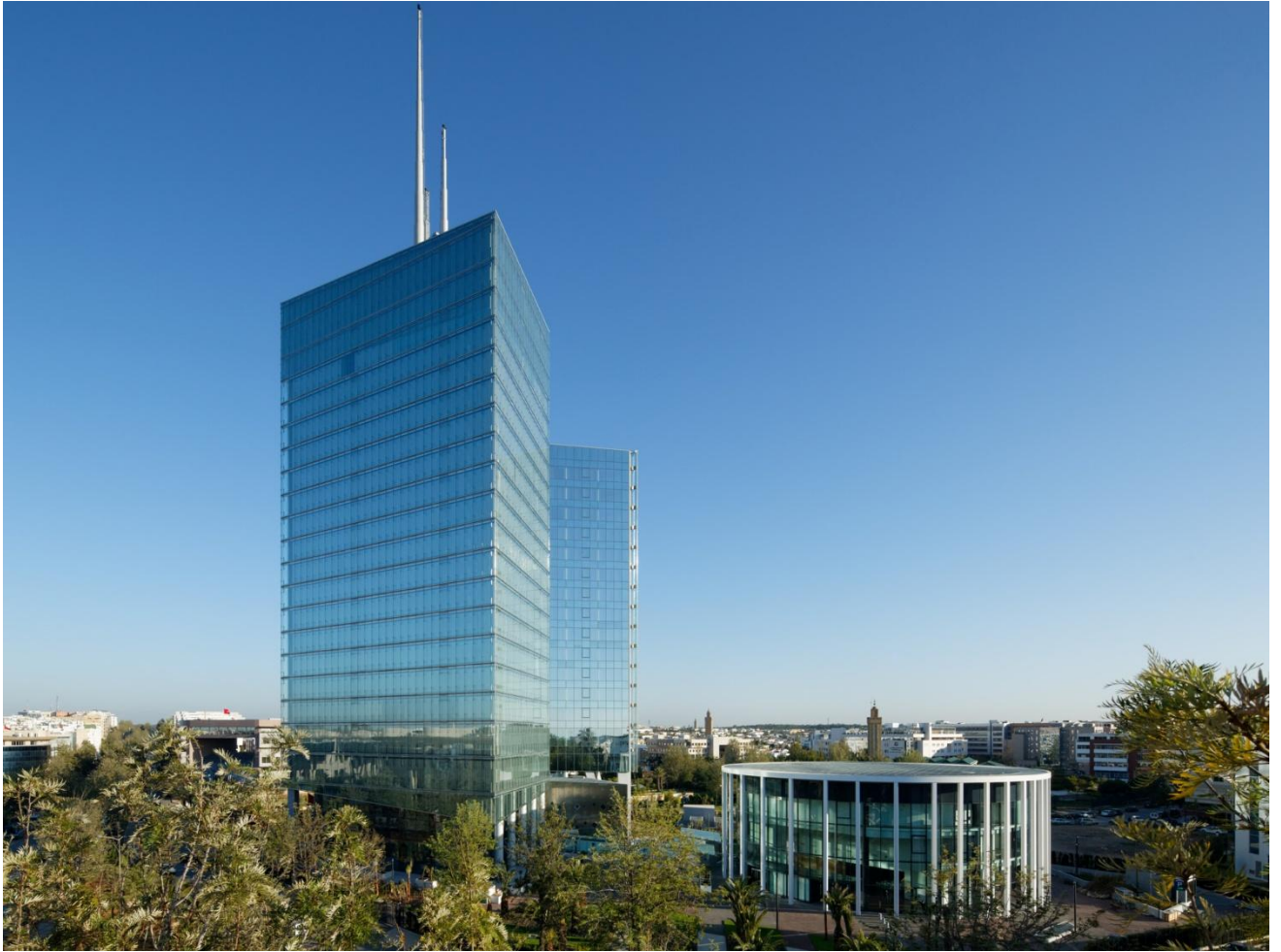
Fig.4.3.2: Maroc telecom headquarter (collected)
