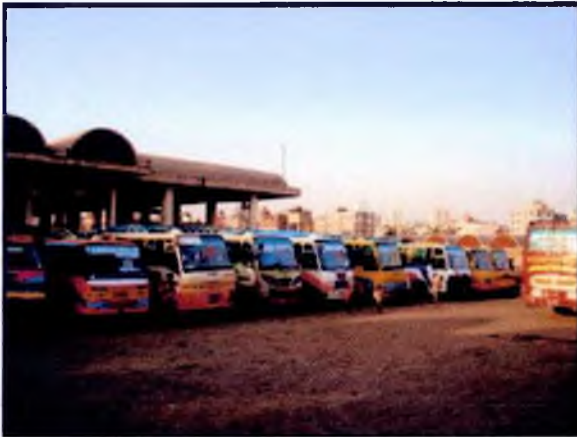
Fig 50: Bus parking under canopy Source: www.panoramio.com
