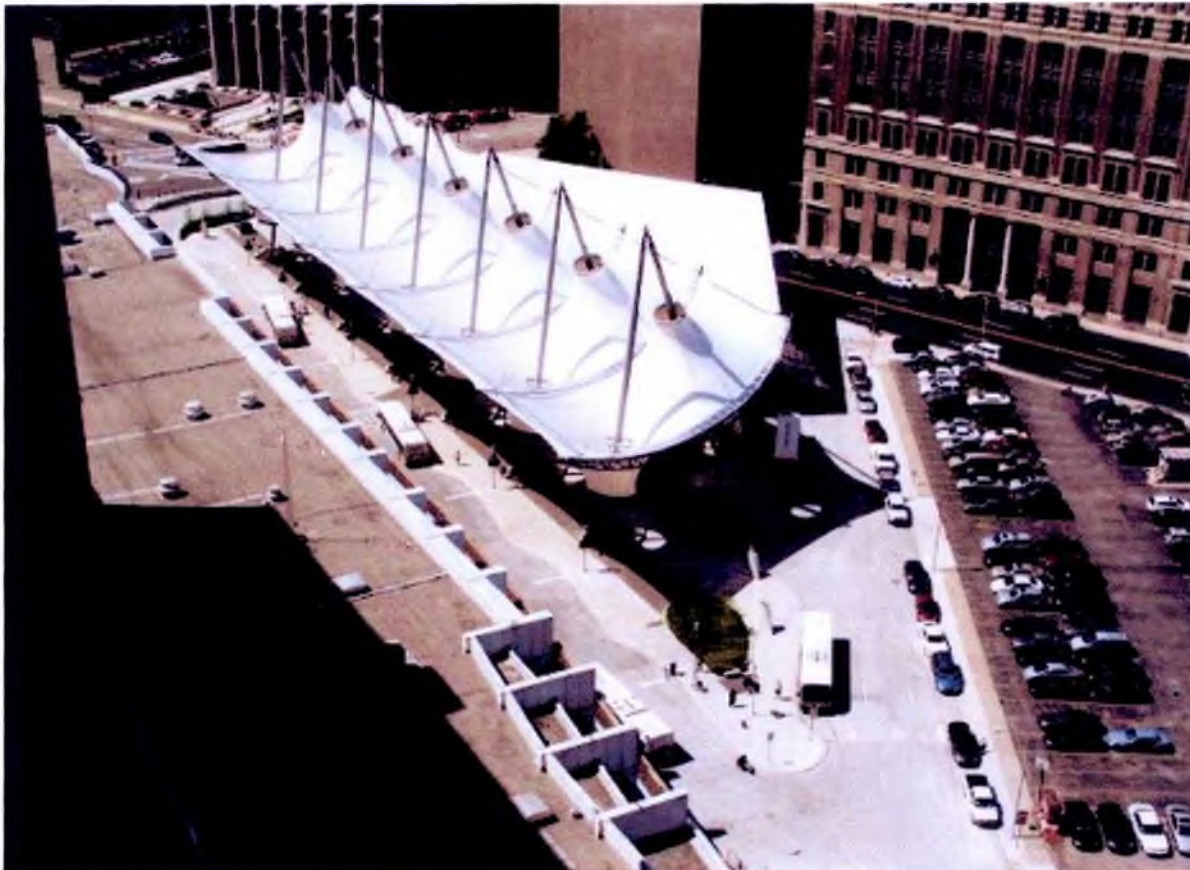
Fig 28: View from top Source: www.archdaily.com
