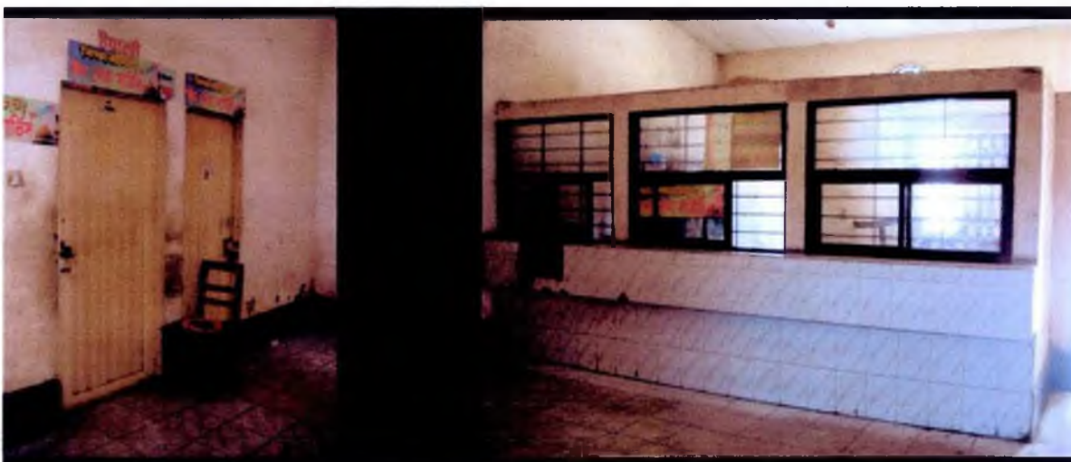
Fig 10: Existing Toilet facility Source: Hoque, 2011
