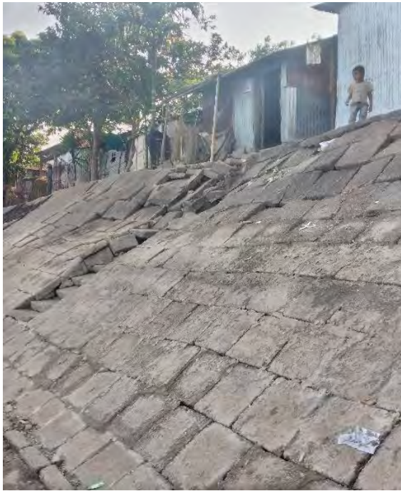
Fig-40: Blocks displaced by floodwater
