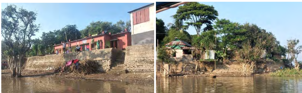
Fig-44: Brick protection wall of Anondonagar
