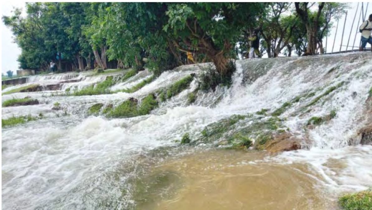
Fig-23: Floodwaters overflowing an embankment in Tahirpur upazila, Sunamganj in 2022. (Star, 2022)
