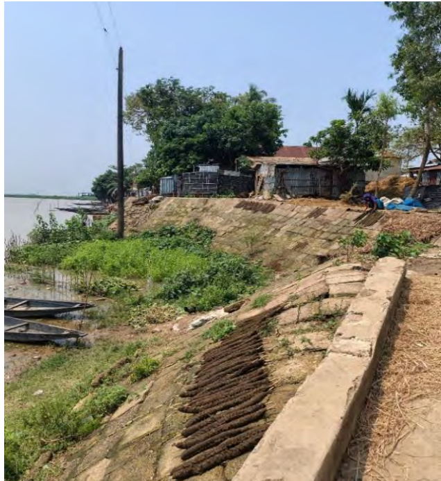
Fig-41: Protection wall by concrete blocks
