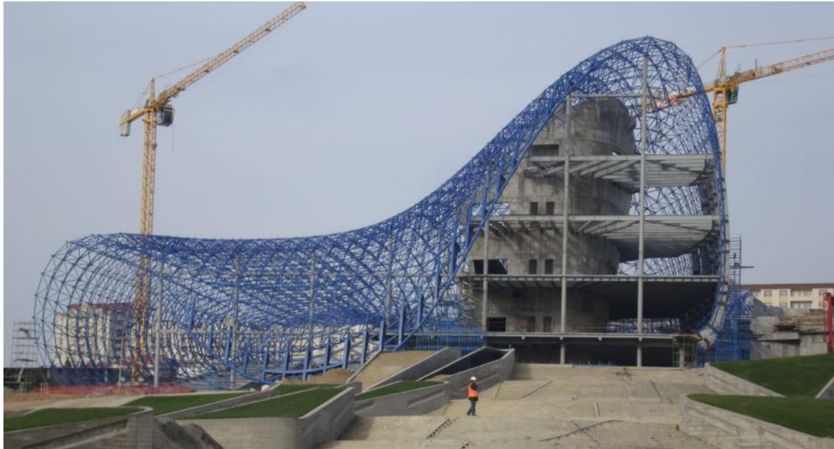
Figure 15: Construction of Heydar Aliyev center (Source:buildipedia.com)
