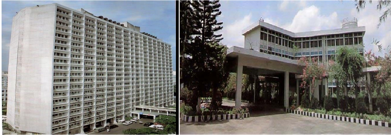
Figure 4.2: Some important projects of PWD (at the left- the national secretariat building, at the right- the public administration training academy)
