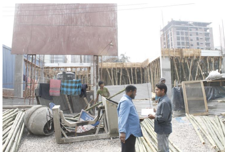
Building Under construction for shop
