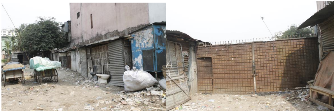
One of the few store house,view from inside and outside of the gate
