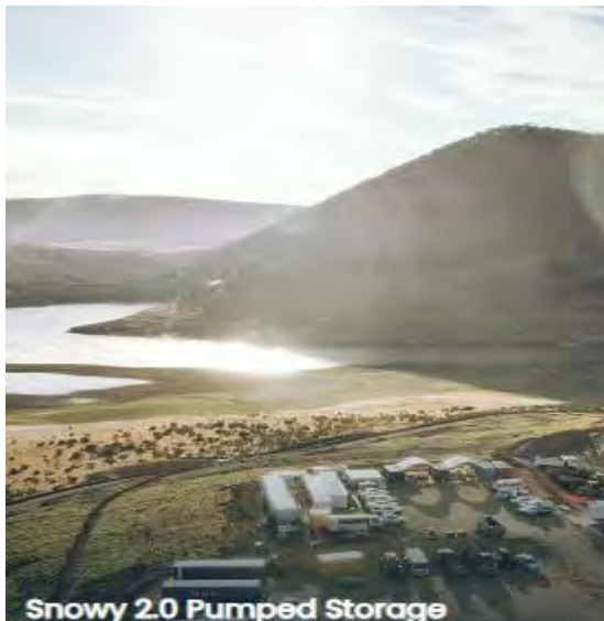
Figure 1: SMEC International Snowy 2.0 Pumped Storage, Australia
