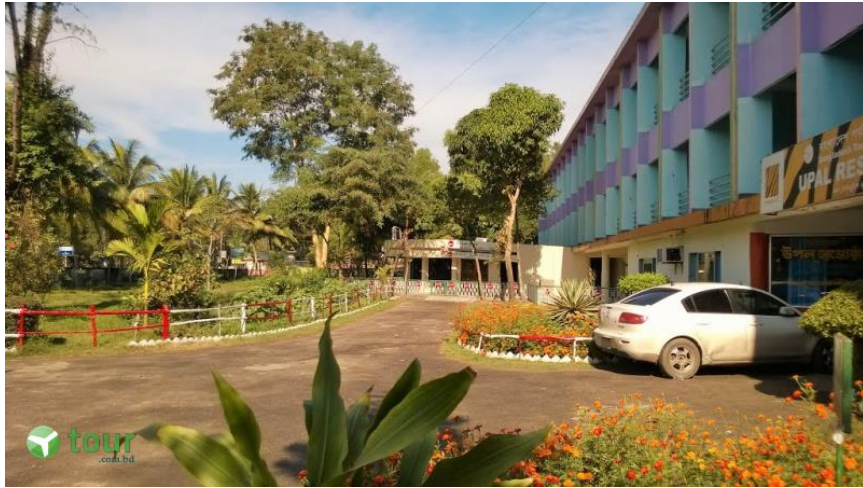
Figure 10: image from south side showing existing landscaped green
