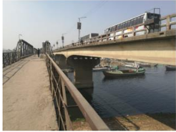
Old Bridge on the left and New Amin Bazar Bridge on the right
