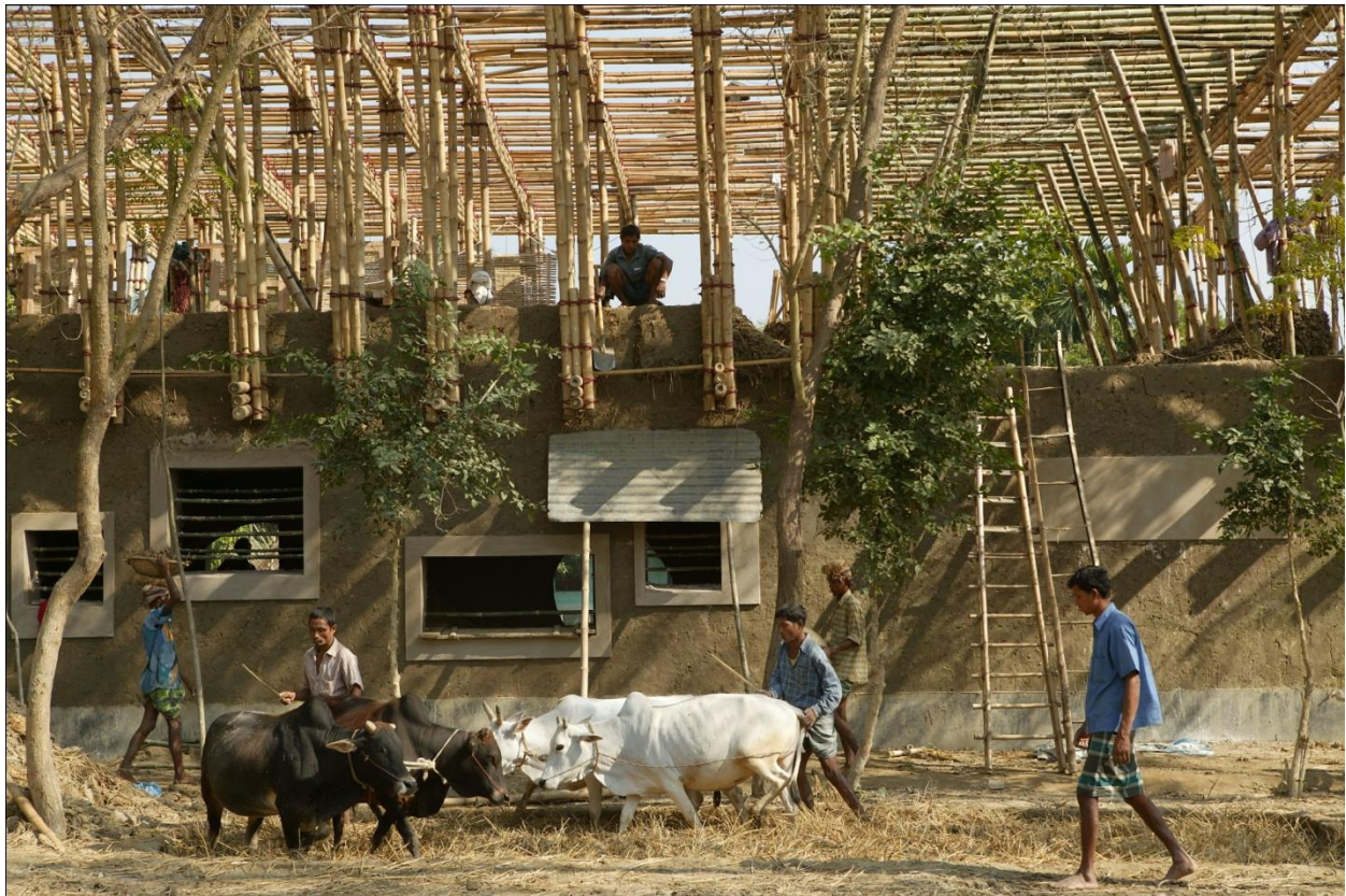
Fig 2.14: METI School under construction Source: Gessato official website (2011) (Retrieved: 28 th July 2016)
