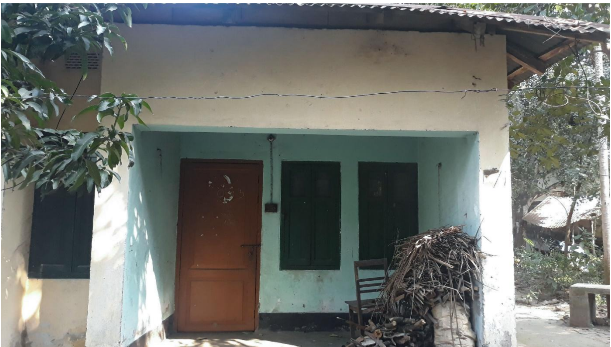
Figure 3.14: Existing staff quarter
