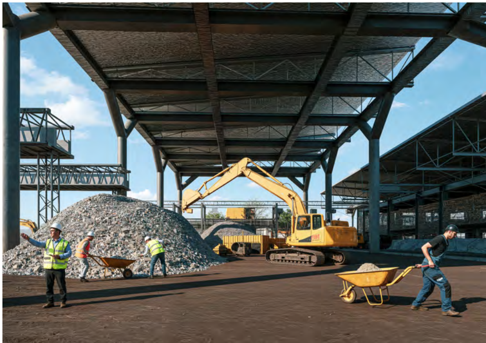
Figure 7.9: View inside shaded Coal yard (Source: Author)
