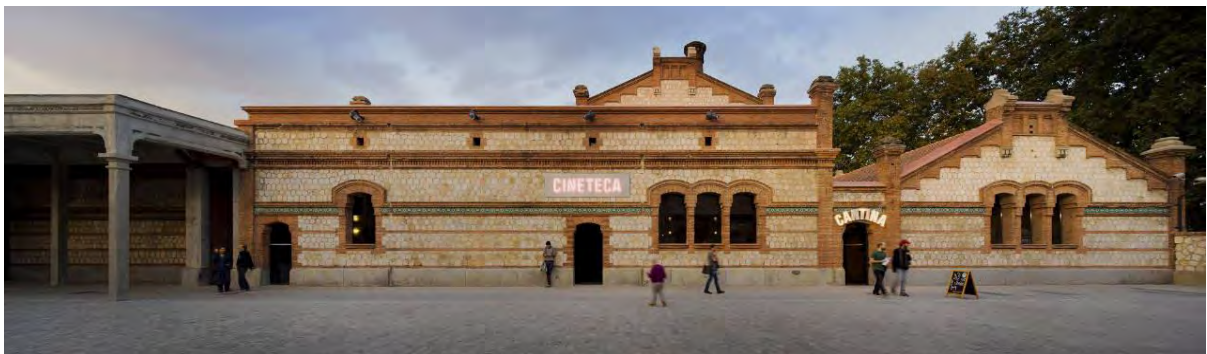
Fig 4.16: Cinema Center in Matadero de Legazpi outer facade (Source: Fernando Guerra | FG+SG, archdaily.com)
