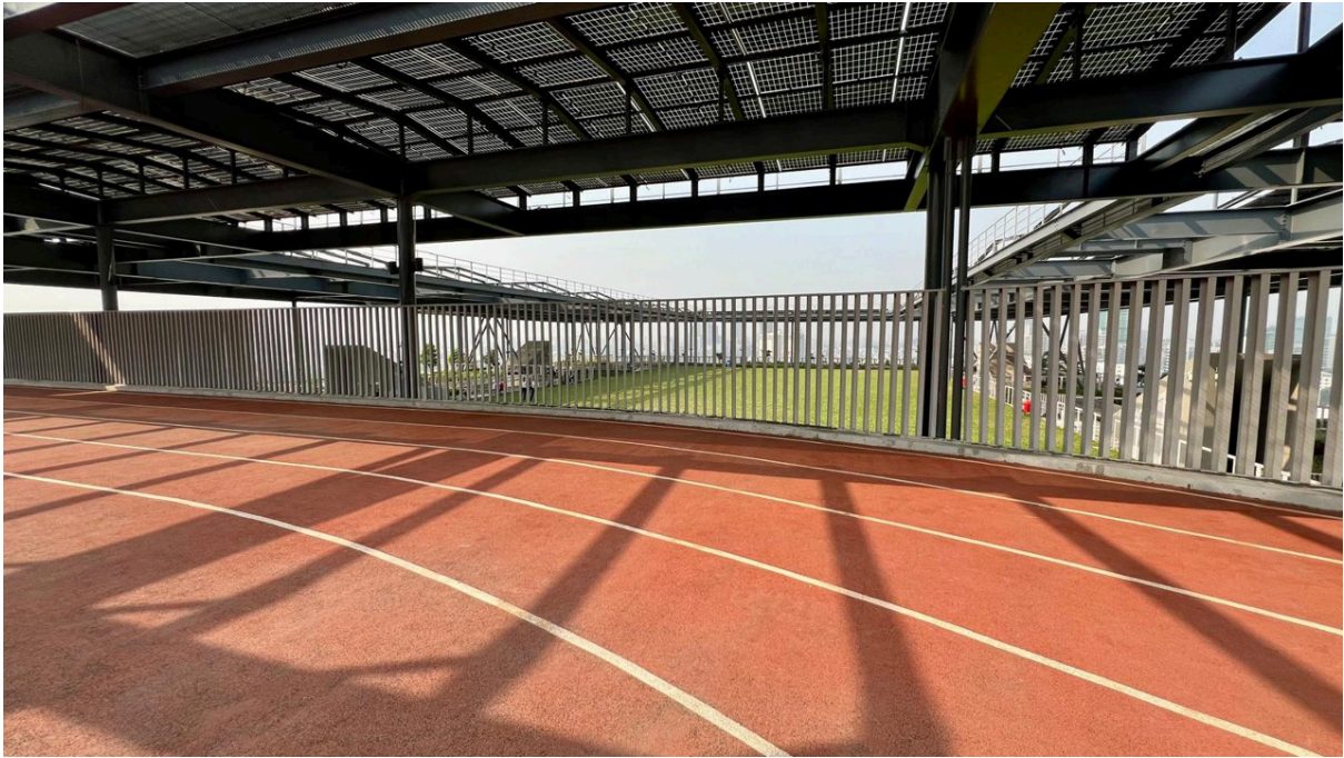
Figure 4.1.K: Running Track of Brac University (Source: www.transsolar.com )
