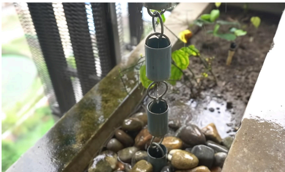
Figure 4.1.N: Rain chain Irrigation of Brac University (Source: author)
