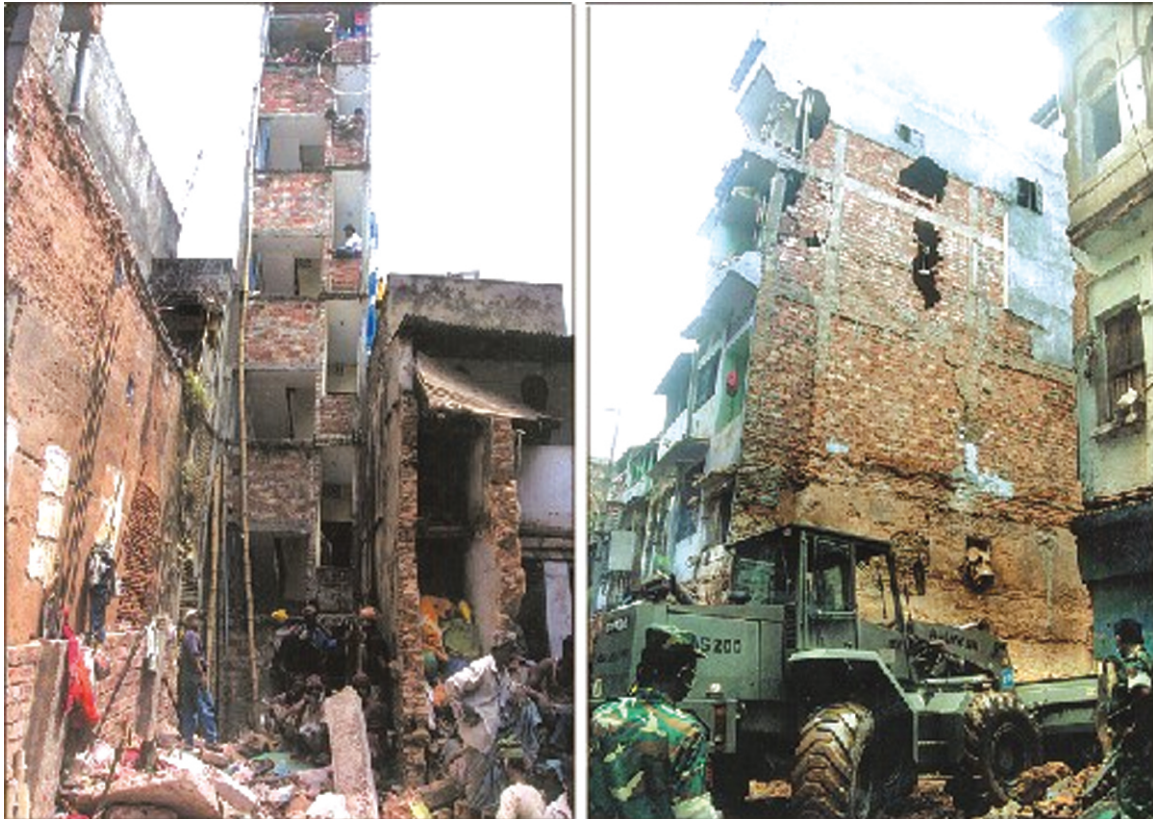
Figure 8: The collapsed house of Shankharibazar Source: The Bangladesh Observer
