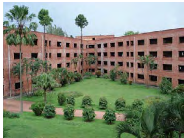
Fig. 3.3 View of the inside
