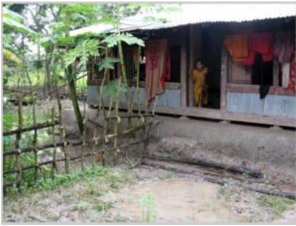
Fig. 4: wooden column in a traditional house
