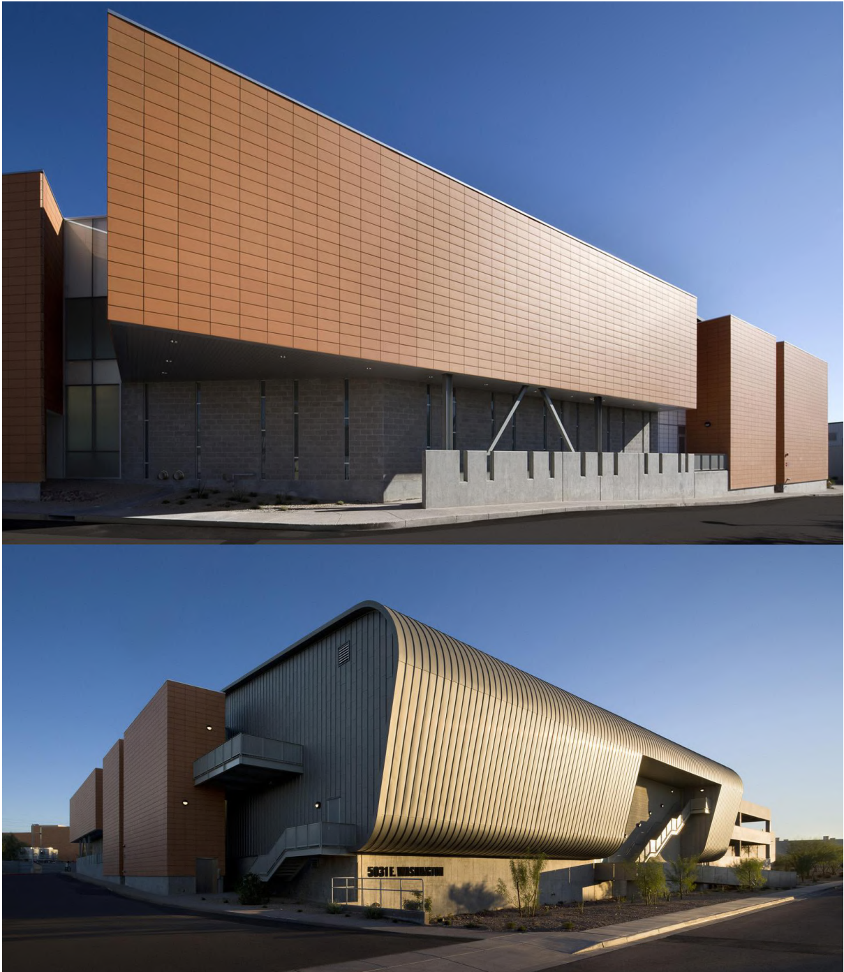
Fig 44: Exterior Cladding (Source: Archdaily)
