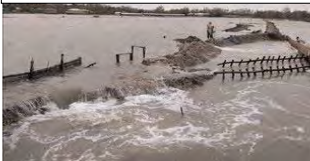
Picture-22: Flash Flood
