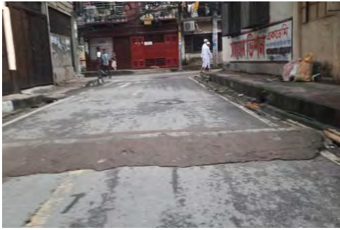
Figure 5.17: Concrete Speed Bump
