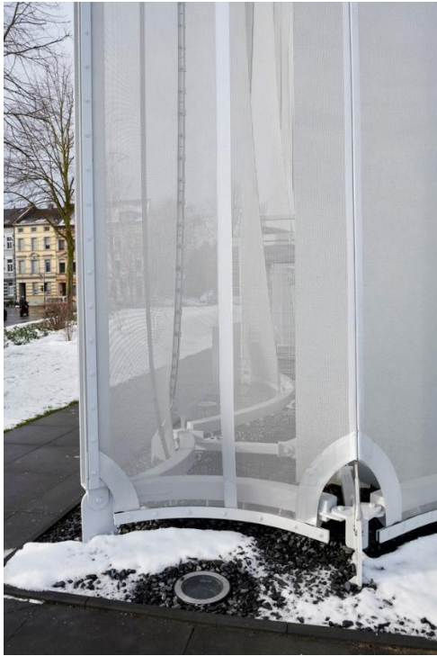
Figure 4.3 7: Curtain fabric installed with steel structure.
