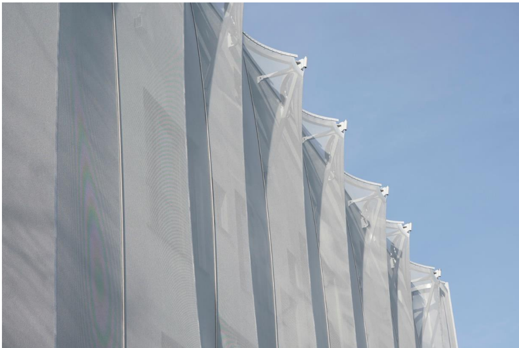
Figure 4.3 8 Fabric fenestration installed with wall
