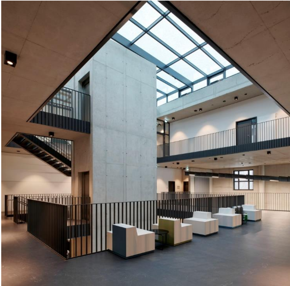
Figure 4.3 4: Stair and core in the middle of the form which holds all up.
