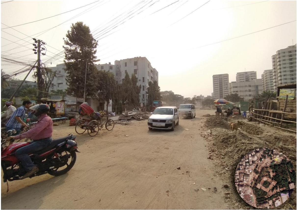
Figure 13 ( showing the newly constructed road, source: author)
