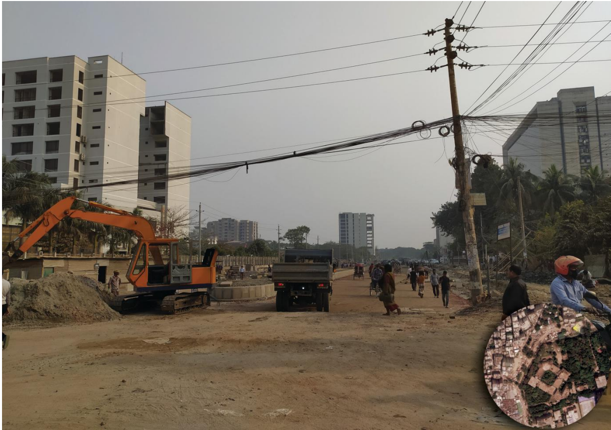
Figure 14 ( showing the newly constructed road and Nuclear centre on the left , source: author)
