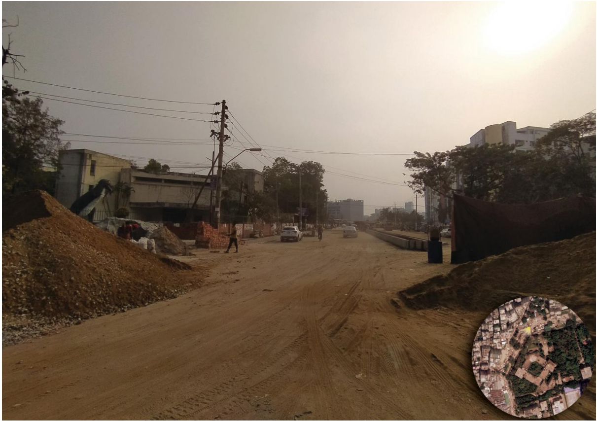
Figure 15 ( showing the newly constructed road and Museum on the left , source: author)
