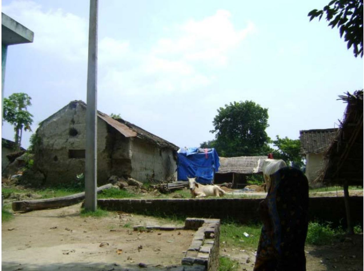
Figure 31: House Being Built On Elevated Plinth and Cemented Boundary
