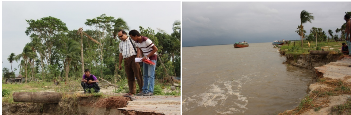
Figure 32: River maintenance and erosion control Intervention
