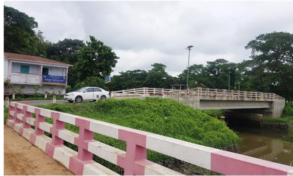
1. VIEW OF CTG-RANGAMATI HWY AND THE EXISTING THANA
