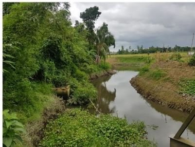
3. EXISTING CONDITION OF THE KHAL THAT FLOWS ALONG THE WEST OF SITE
