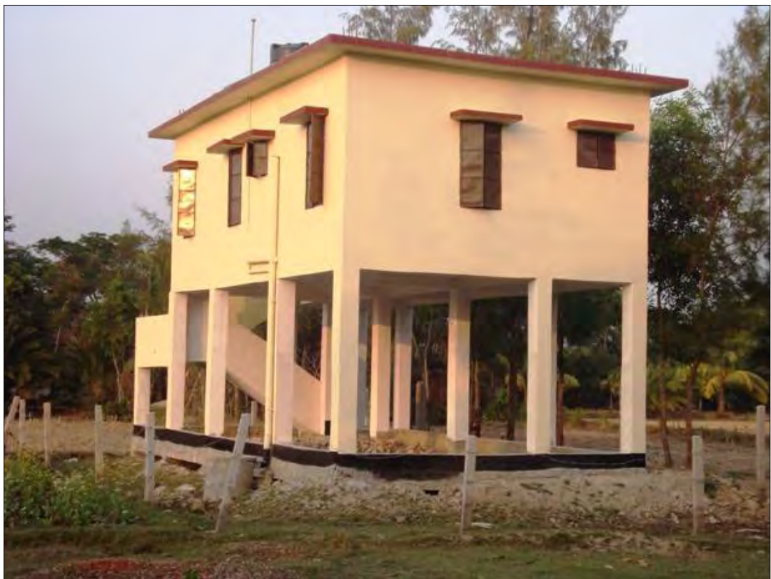
Photo 4.2: Medical centre is under construction near Namar Bazaar, Nijhumdwip (Taken in February 2015)
