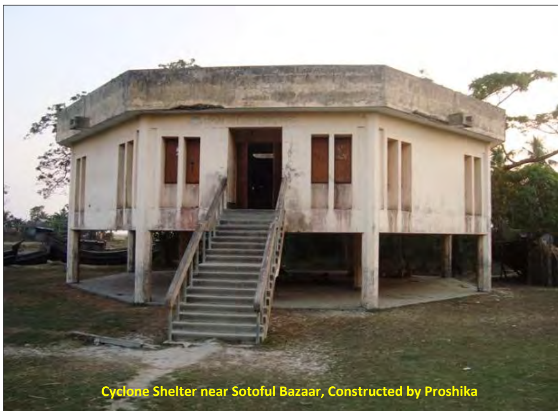
Photo 5.1: Cyclone Shelter constructed by Proshika, Source: Photo taken February 2015 during
