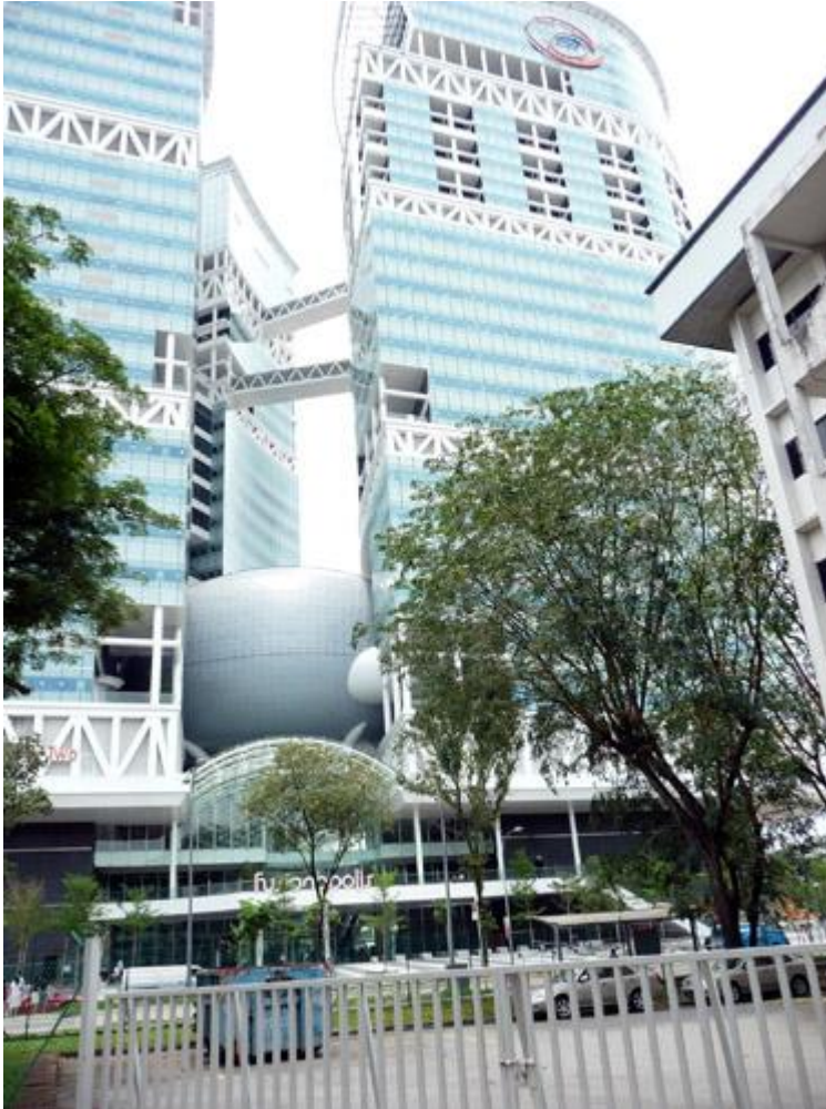
Fig 4.3.2: exterior view of the auditorium
