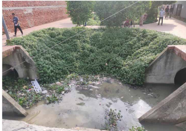
Figure 7 | The sluice gate (Field survey 2022).
