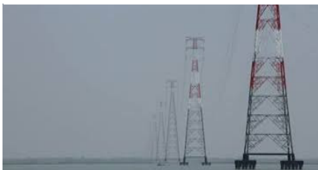
Figure-4: A long HV Transmission Line over a River in Bangladesh
