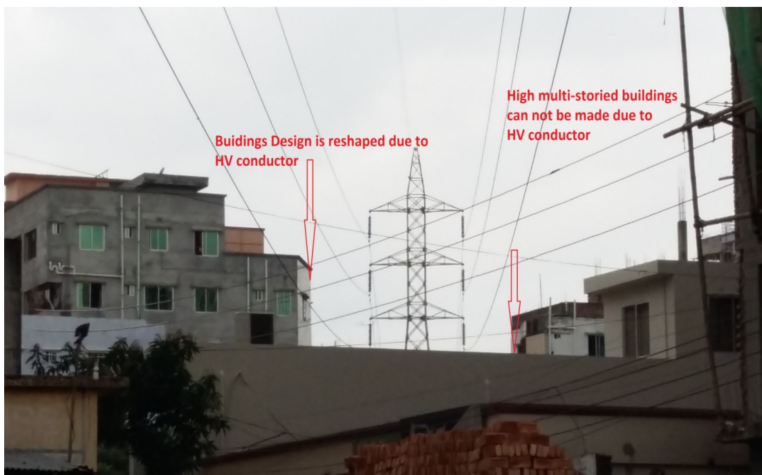
Figure-15: Public/Social/Civil problems created by HV Transmission Lines, causing public dissatisfaction
