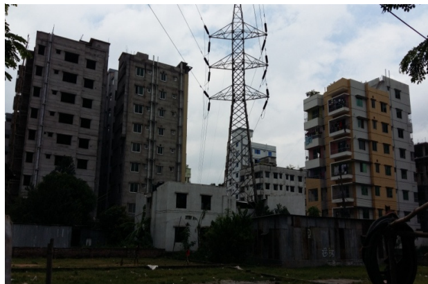
Figure-7: HV Transmission Line and Tower in a Densely Populated Area in Dhaka
