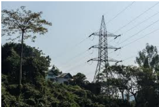
Figure-5: Transmission Line causes deforestation; green trees are cut for the path of clearance
