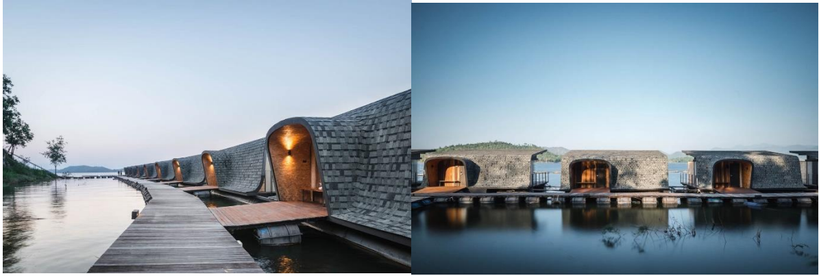
Image 5: Curvilinear roof of the resort
