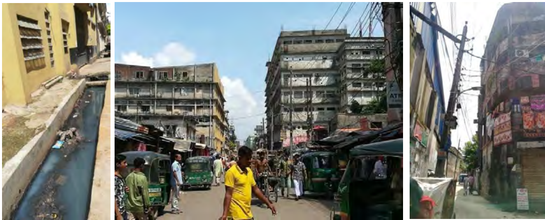
Fig.3.3.2. Road conditions in the area
