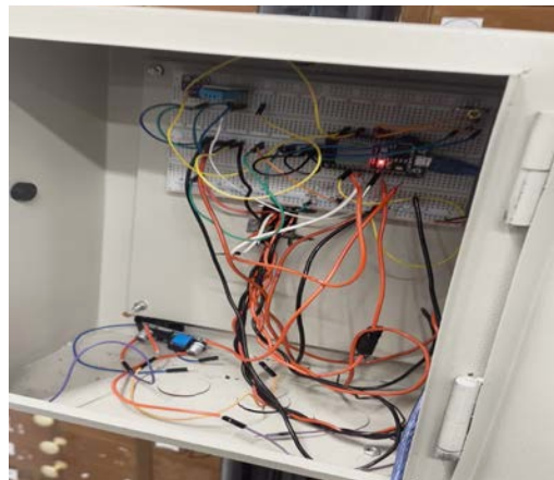
Fig 5.2.5.1- IP67 - rated waterproof box for circuit sheltering
