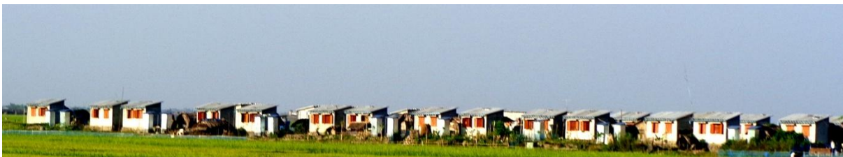
FIG: 4.9 Disaster resilient Bainpara village, union Sutarkhali under the Dacope upazila of Khulna district, 2012
