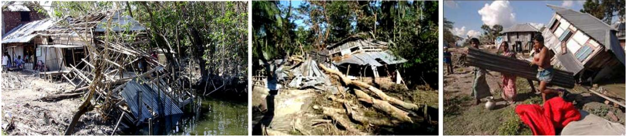
FIG: 2.3 Pictures Illustrates of the Damage by Cyclone Sidr in Bangladesh.
