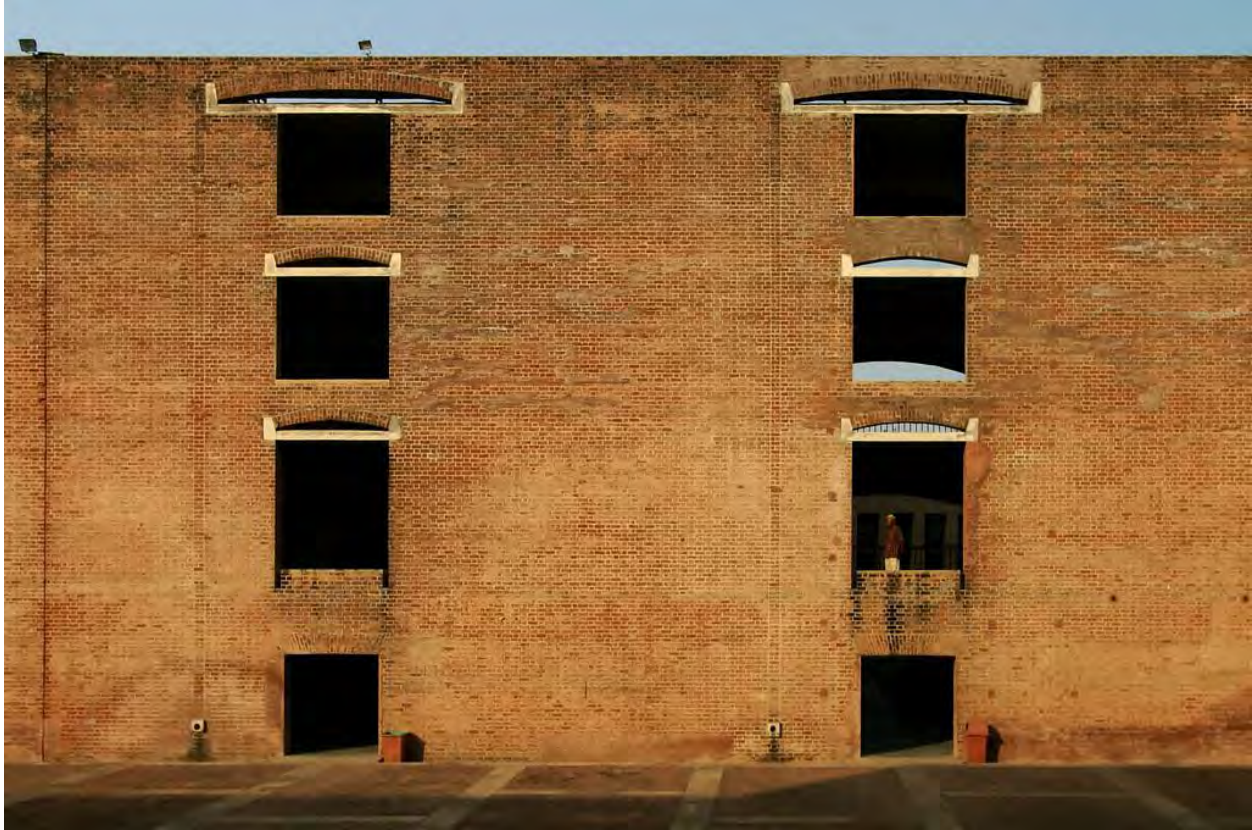
Figure 4.4.d: IIM University campus façade detail. Source:
