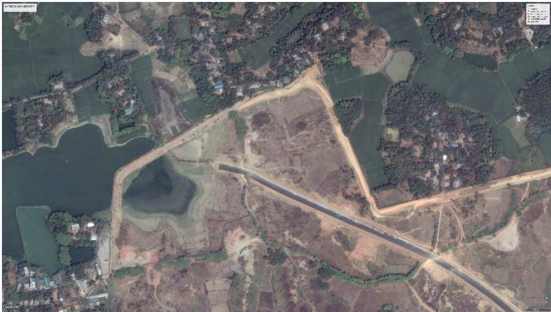
Figure 3.6.c: Satellite view at March. Source: (Google earth pro gold satellite view)
