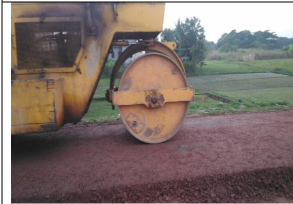
4. Compaction work of base course.
