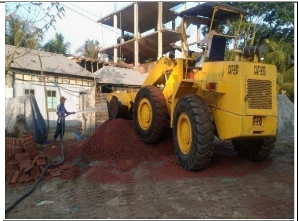
2. Mixing & watering of base course.
