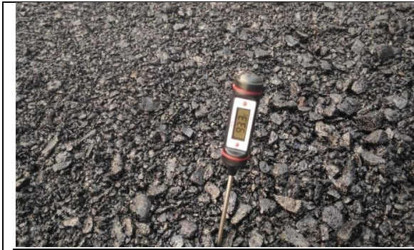
8.Rolling temperature checking
