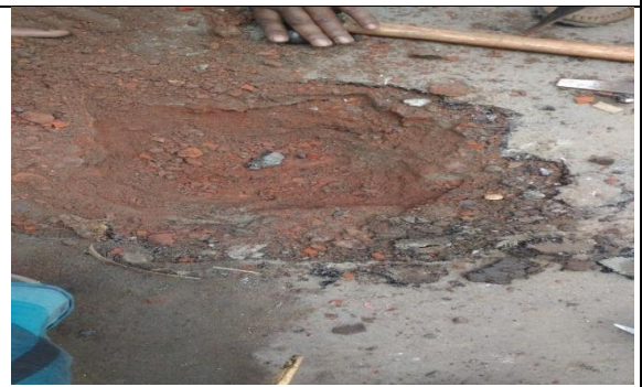
13.Post thickness checking of all layers of road.
