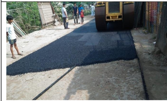
12.Using PVC pipe for proper thickness
