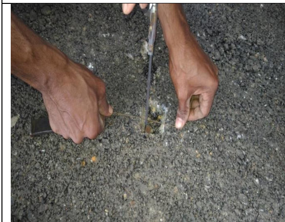
6. Thickness checking of BC work
