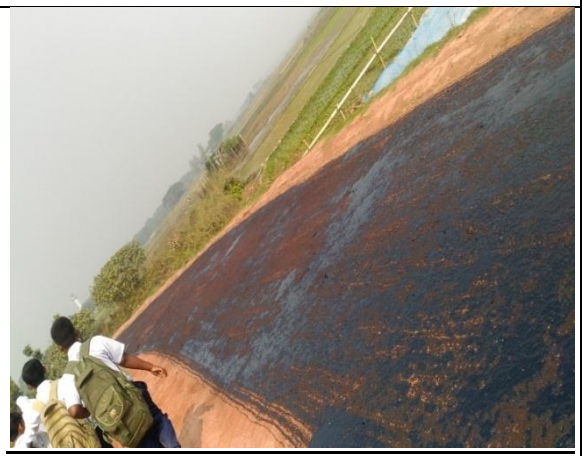
7. Prime coat work ongoing.
