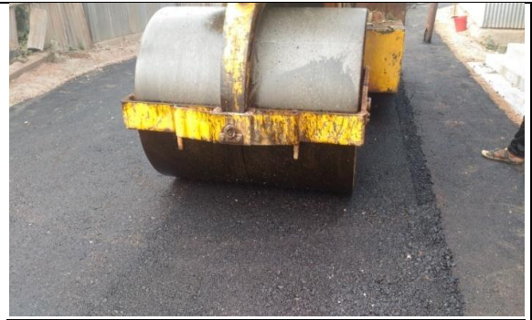
9.Compaction work ongoing of BC.
