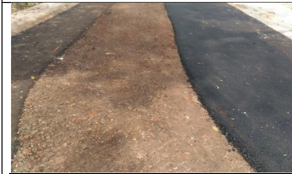
10.12mm Seal coat work ongoing.
