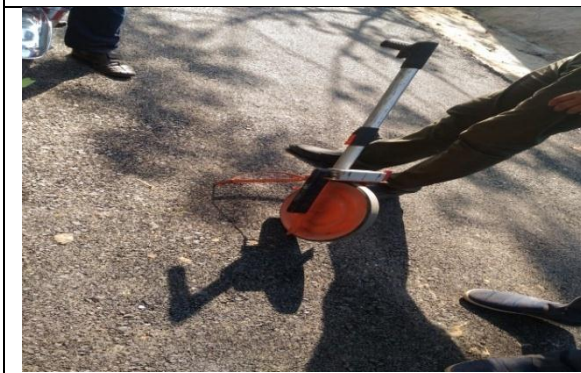
14.Using Distance wheel for measuring length of road.
