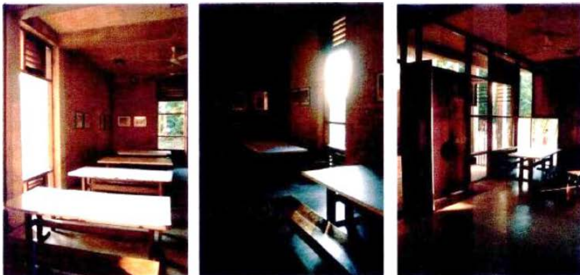
Fig.4.2.d. Classrooms, Good ventilation and Natural Lighting (Tahseen, 2012)
