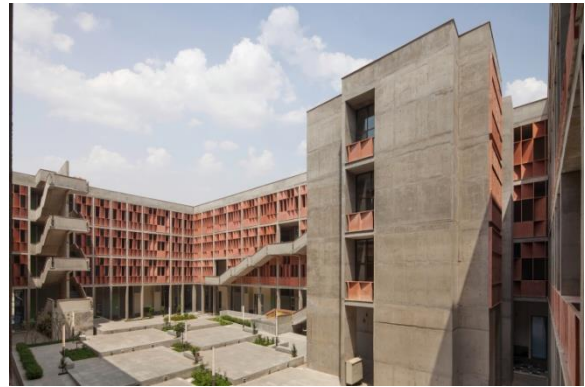
Fig 4.1 1 View from courtyard (source:virmueller.com)
