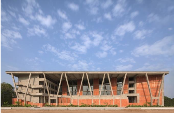
Fig 4.1.2 Exterior view (source: virmueller.com)
