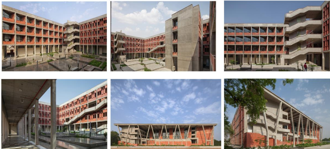
COURTYARD SAND BRICK FACADE PATTERNED FACADE PROVIDE POCKETS OF INSULATION OF AIR THE USE OF CONCRETE, GIVES A COOL COLOUR AGAINST THE HOT TEMPERATURE NATURAL LIGHT
