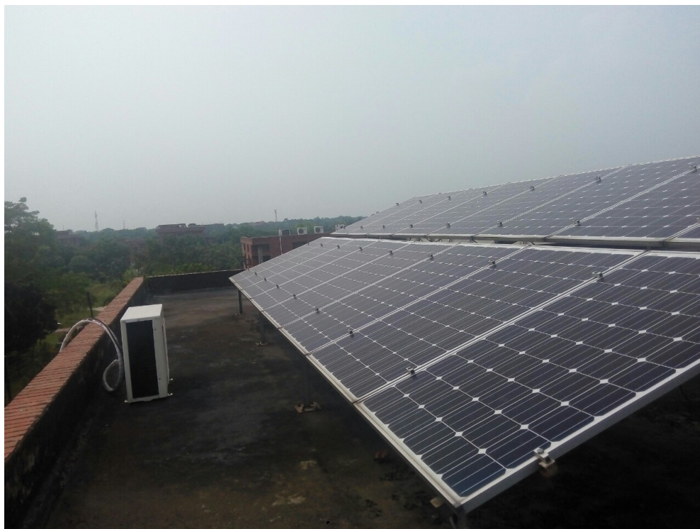
Figure 4.2: PV Array Side View
