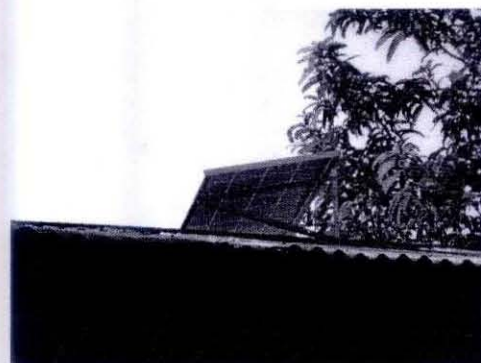
fig 4.6: solar panel (source Author)
