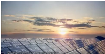
Solar panels on the roof
