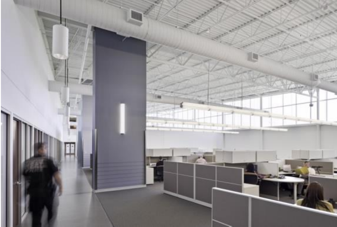
Diffused natural light pervades the work areas of Lancaster Public Safety Facility.
